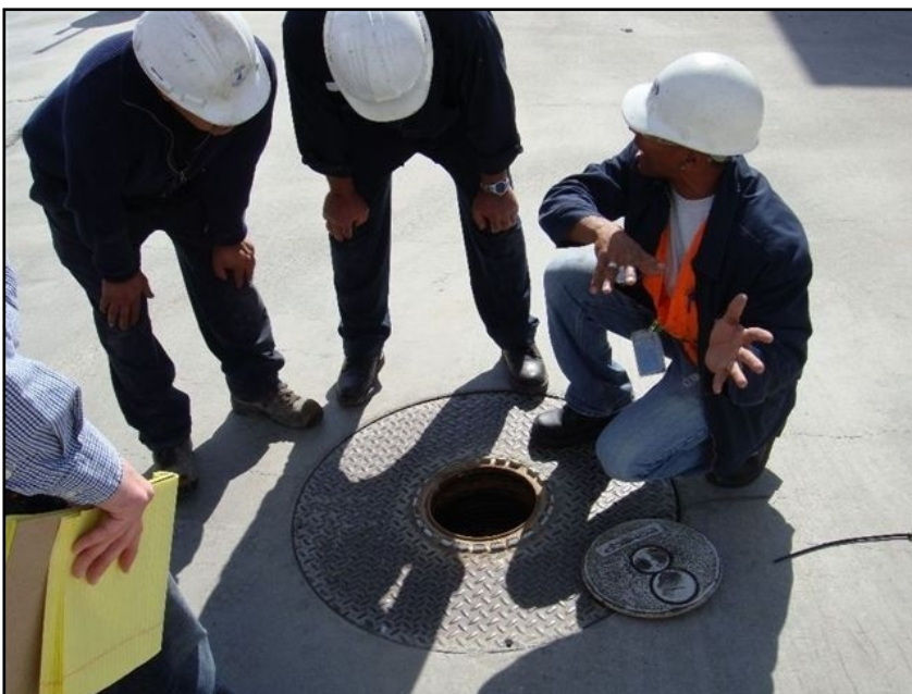
Photo of UST port inspection courtesy of Orange County CUPA
